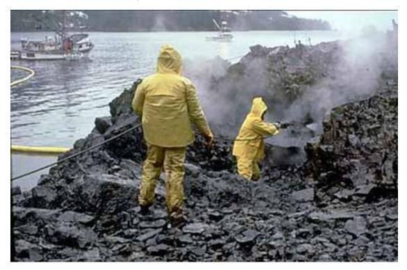
A brown sediment plume and sheens of refloated oil drift away from this oiled beach as it is cleaned by a team applying highpressure, hot-water washing. Refloating of oil and release of sediment are often unavoidable consequences of shoreline cleanup that can cause additional environmental harm.
